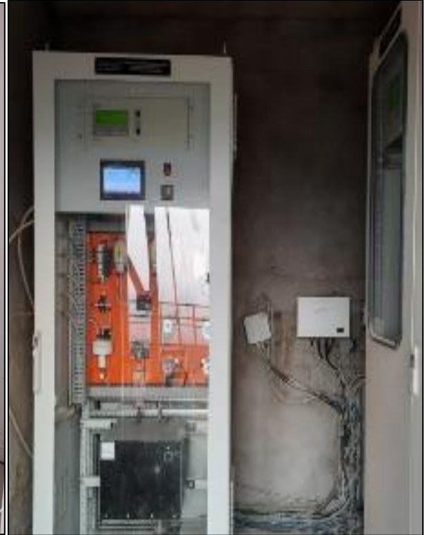
Installation of CEMS for Gaseous Emission Monitoring at Raw Mill + Kiln and CPP
