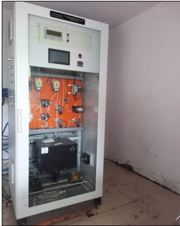
Installation of CEMS for Gaseous Emission Monitoring at Raw Mill + Kiln and CPP
